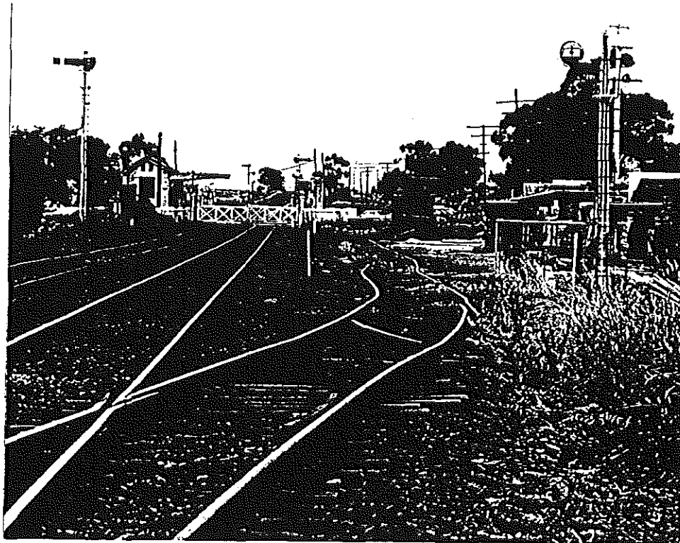
Site of Sydenham chaff-mill, 1987. Now occupied by a garden nursery, note the siding in the foreground. Photo. G. Vines.
