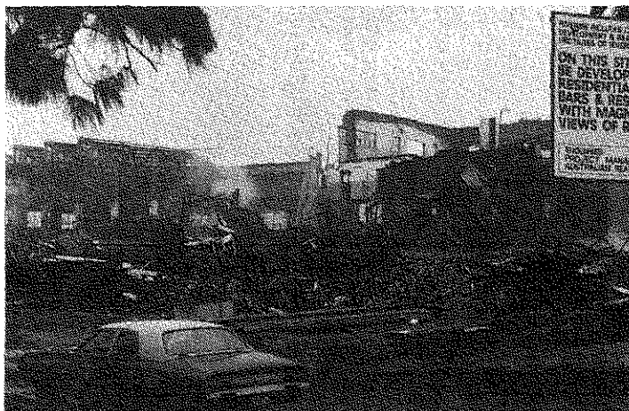
Demolition of the Michaelis Hallenstein Tannery in Footscray, 1987
