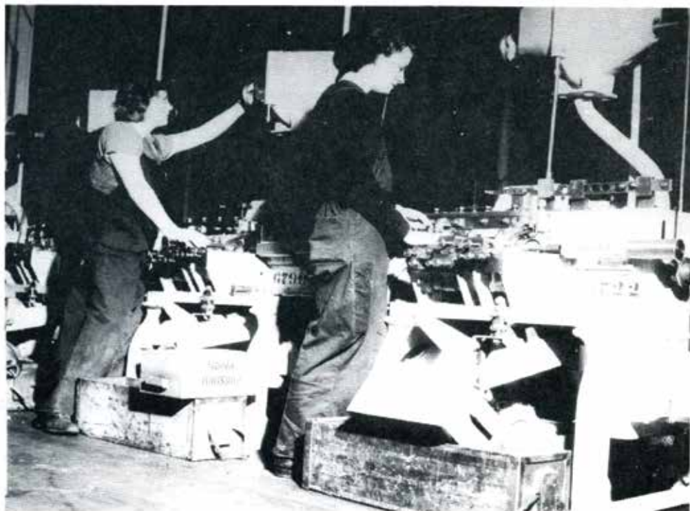
Turning Heads of 9 mm cartridge cases on automatic lathes, Gordon Street.
