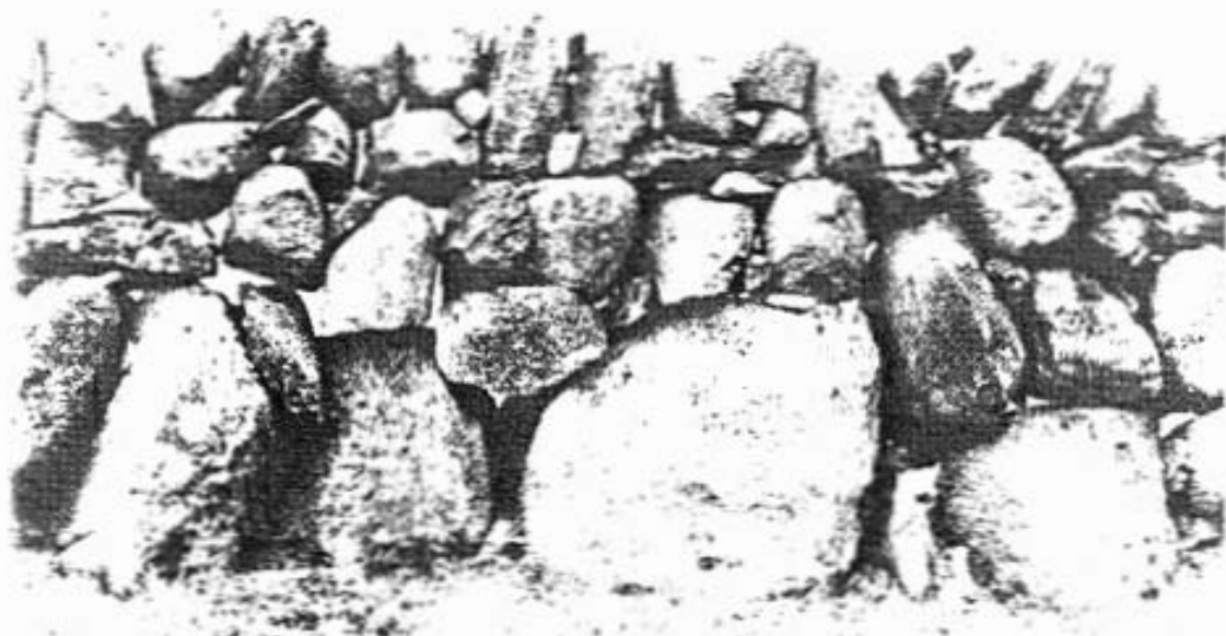
Plate 2. Example of "single" wall common in the Galloway district of Scotland.
