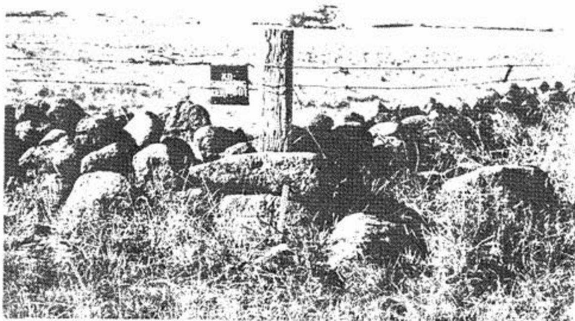
Site No. 003 Detail of Wall Head and Corner Stones
