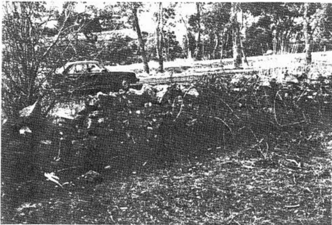
Plate 6. Stone Wall built from sandstone near Chewton, Victoria.
