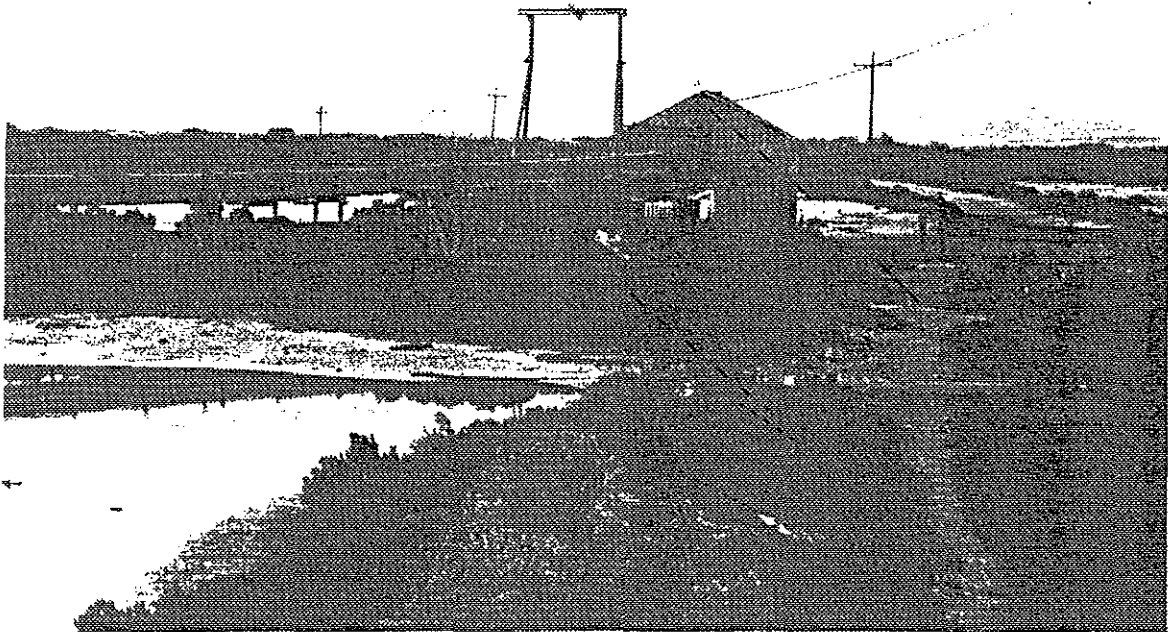
35. No. 2 pump house and timber chanelis
