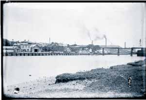
The view from across the river to Maribyrnong Street during the 1920s when the Bunbury Street rail bridge and tunnel were under construction. Footscray wharves line the waterfront. The Ship Inn is on the left. In the background smoke belches from the Michaelis-Hallenstein tannery. PROV, VPRS 12800P7, Public Transport Corporation Photographic Collection, C/0315. Reproduced with the permission of the Keeper of the Public Records.
