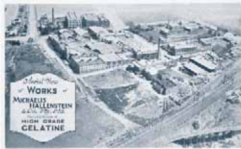
The vastness of the Michaelis-Hallenstein site is shown in this aerial view from 1930. A portion of the Hopetoun Bridge and the Footscray Wharves are captured in the top left corner. Hopkins Street dissects the Michaelis-Hallenstein complex. La Trobe Picture Collection, State Library Victoria.
