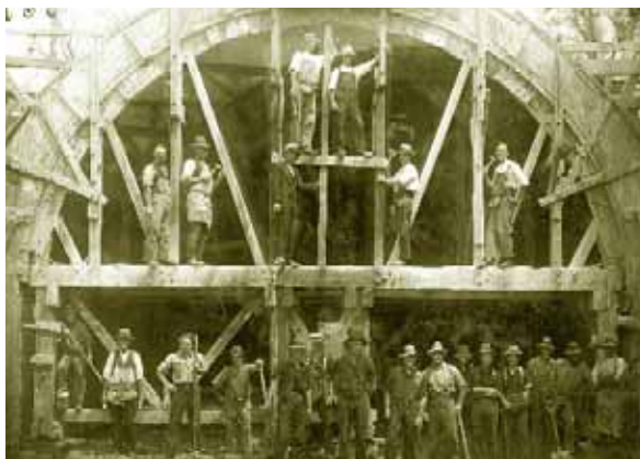
Workers building the Bunbury Street Tunnel in 1928. Photo: Wilfred Disney Chapman. La Trabe Picture Collection, State Library of Victoria.
